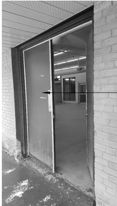
PHOTO 10: REMOVE DOOR, FRAME AND PUSH BUTTON FOR DOOR N-100A
