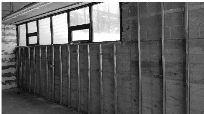
PHOTO 04: REMOVE EXISTING METAL STUDS, FLOOR TILE AND GLAZING UNIT
